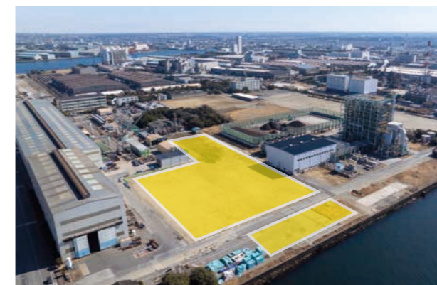
The construction site for the Ichihara Sorting Center
